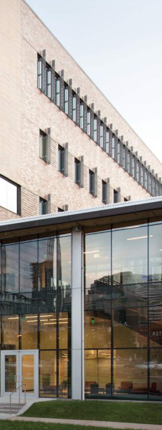
Lynx Center, Colorado University Denver Student Commons Building, Denver, CO. ©BradNicolPhotography, bradnicolphotography.com.
